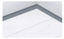
The joint between the rolls should be flush, cut to the required size with a cutter.
