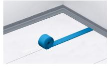
**4.** It is advisable to seal with rough adhesive tape to prevent moisture from entering and with overlapping tape on the edges.
