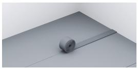
2. Join the sheets together using the Label Tape 70, also apply to vertical and other areas as required.
