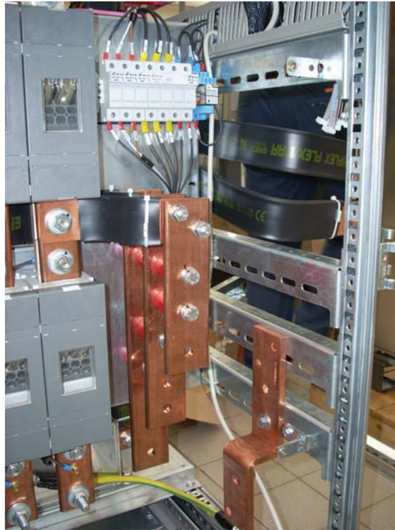
Picture 3 – Position of thermal probe for external battery cabinet for 400...800kVA 3ph-3ph UPS
