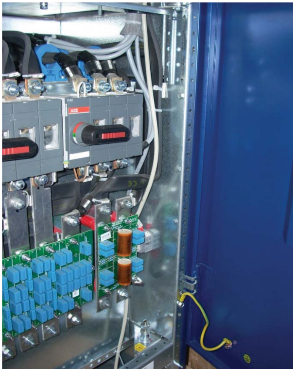
Picture 1 – Position of thermal probe for external battery cabinet for 100...160kVA 3ph-3ph UPS
