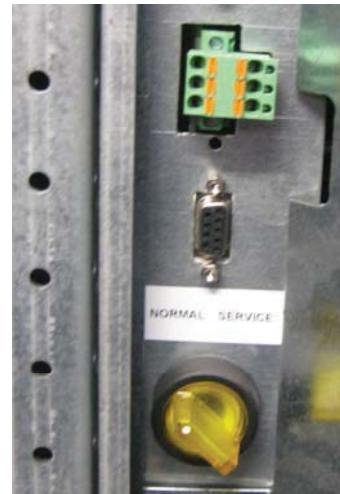
Picture 3 – RS485 Board after the installation (100...800kVA series FXS)
