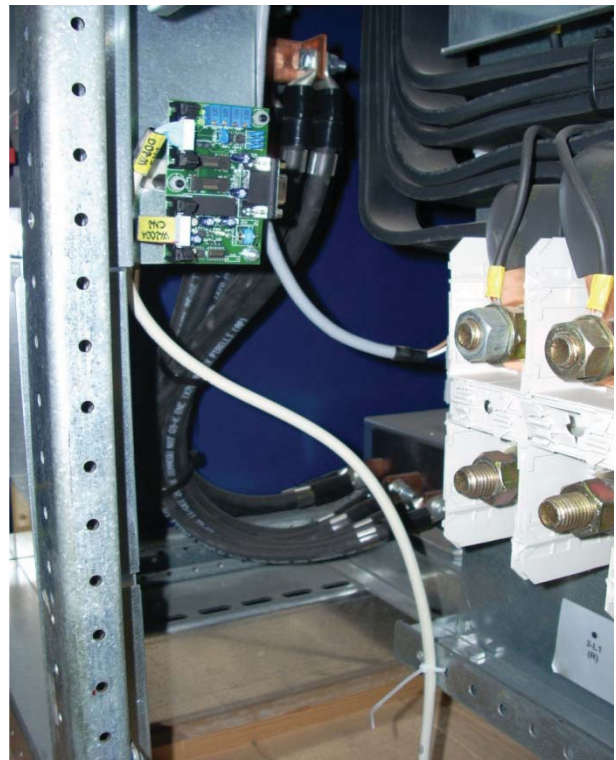
Picture 2 – Position of thermal probe for external battery cabinet for 200...300kVA 3ph-3ph UPS
