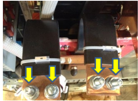
Fig. 6. Removing of the bolts nuts and washers
