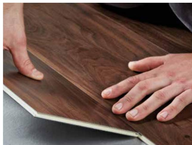
3. No need for adhesive, click and lock the planks into place.
