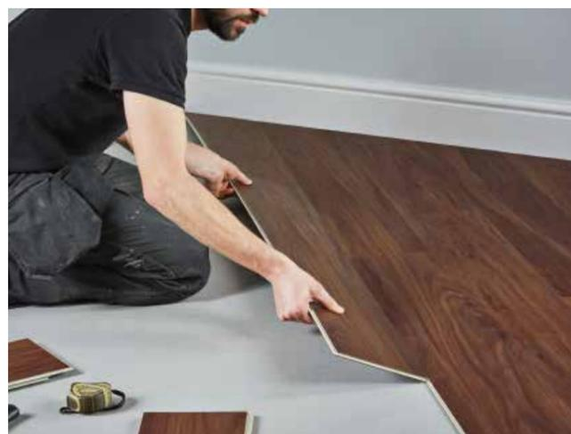
4. Continue to fit the rest of the floor. Remember to leave a 5mm expansion gap.
