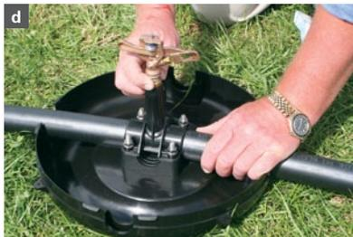
Screw sprinkler into sprinkler riser.
